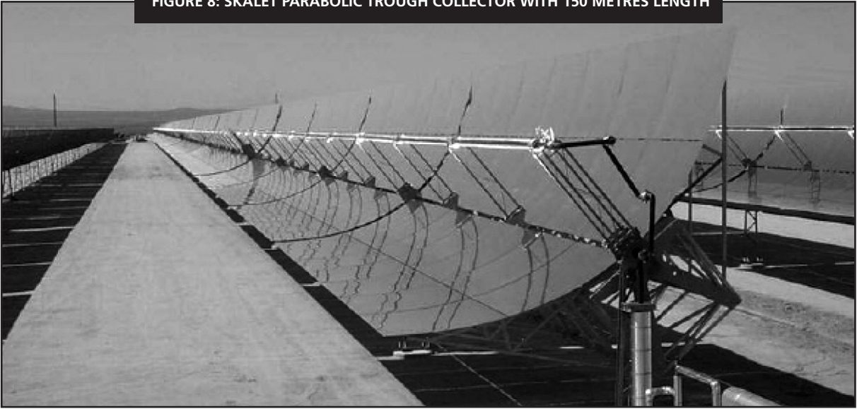
FIGURE 8: SKALET PARABOLIC TROUGH COLLECTOR WITH 150 METRES LENGTH
