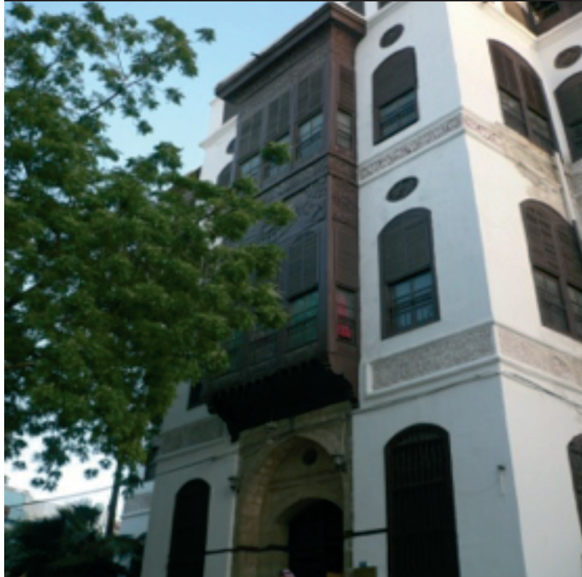
Bayt Nasif, restored façade with mahogany filigree balconies (rawashin, sing. ruwshan), decorative and symbolic elements developed both to respond to climatic needs and to express perceptual identity (author, 2012).
